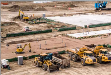
Safe Digging and Excavation Training
