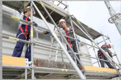
Scaffolding Training for Construction
